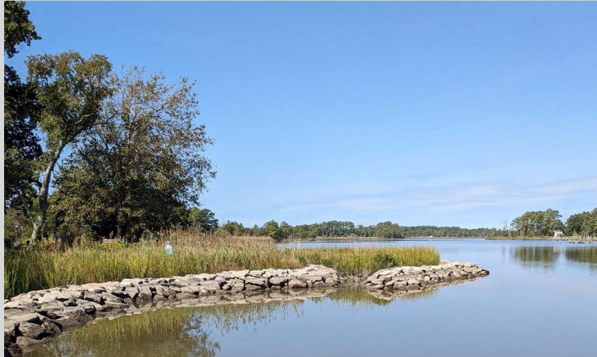
Koontz, E. (2023). View of a gap between the riprap segments at a segmented sill living shoreline in Dorchester County, MD.
